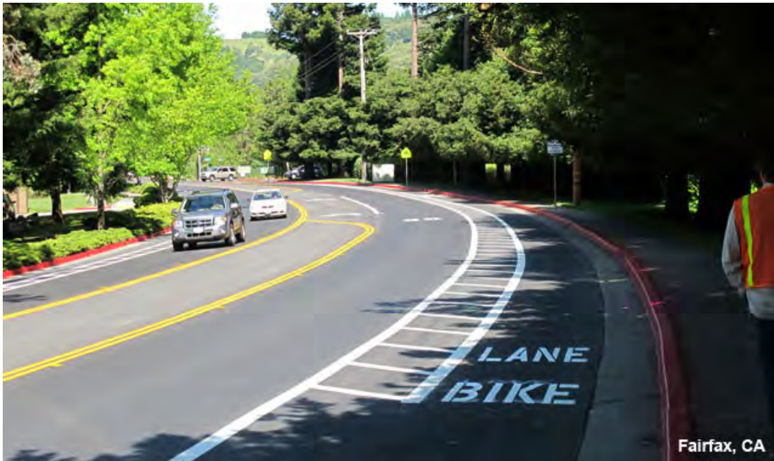
Figure 25. Example of a Buffered Bike Lane (from the NACTO Urban Bikeways Design Guide)
