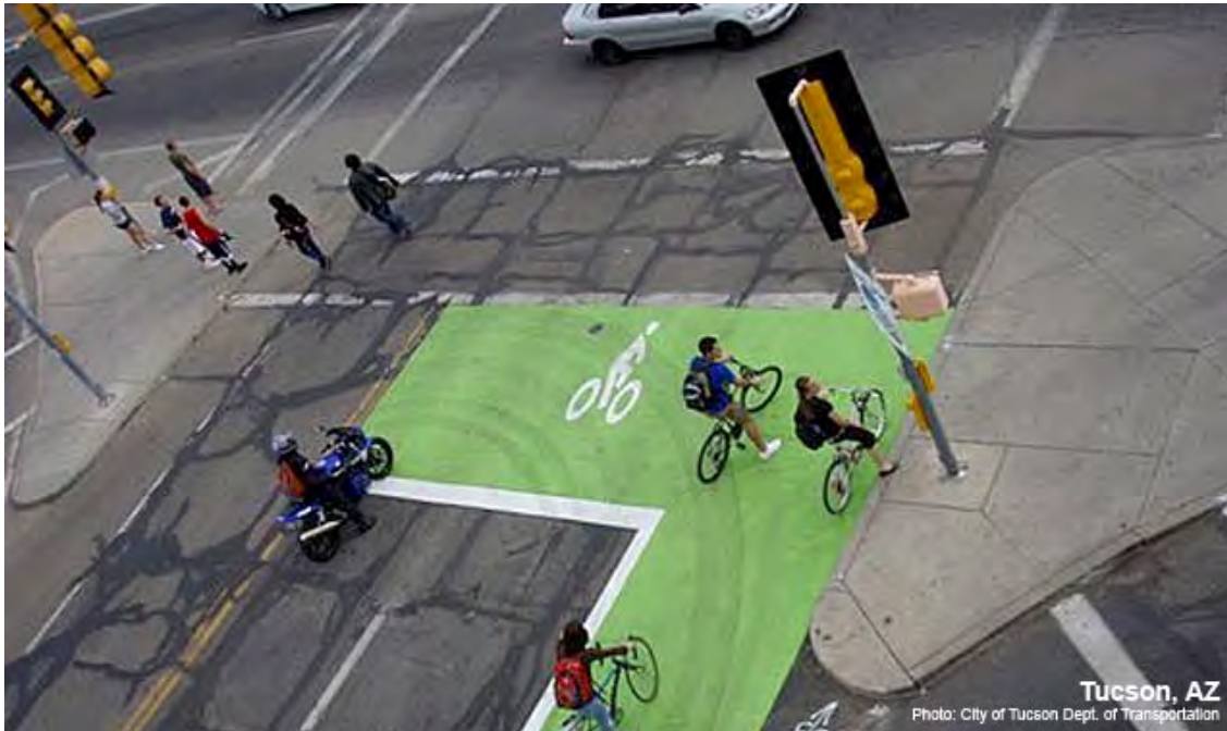
Figure 26. Example of a Bike Box (from the NACTO Urban Bikeways Design Guide)
